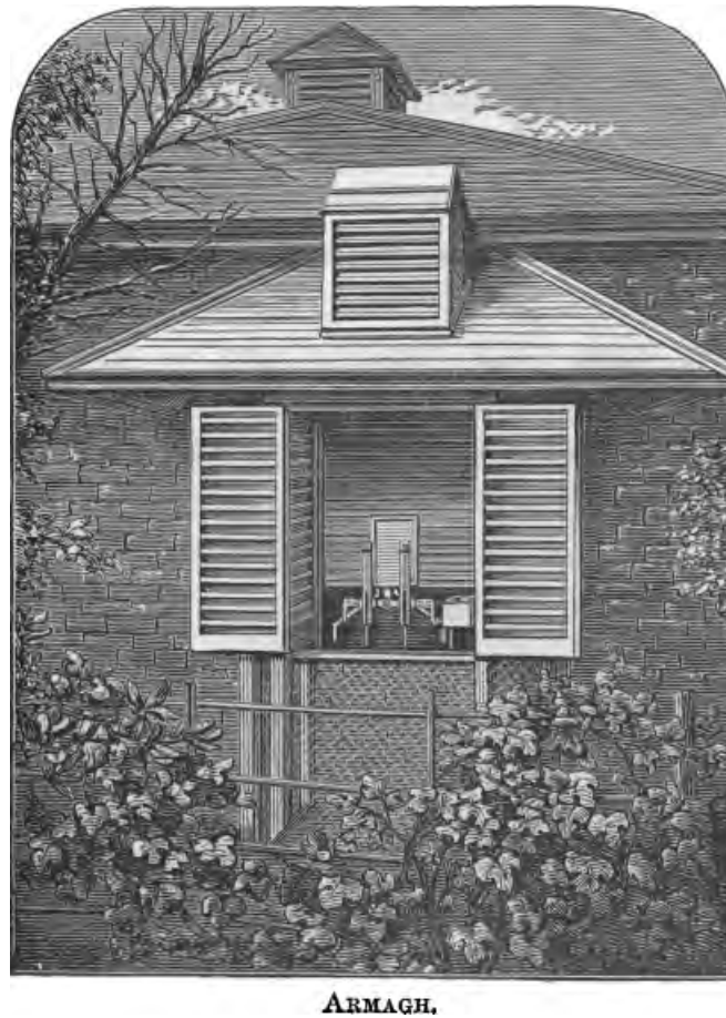
Figure 1. The NWS of the SRT installed at Armagh Observatory by the Board of Trade in 1869. From Quarterly Weather Report of the Meteorological Office for 1870 . HMSO: London
